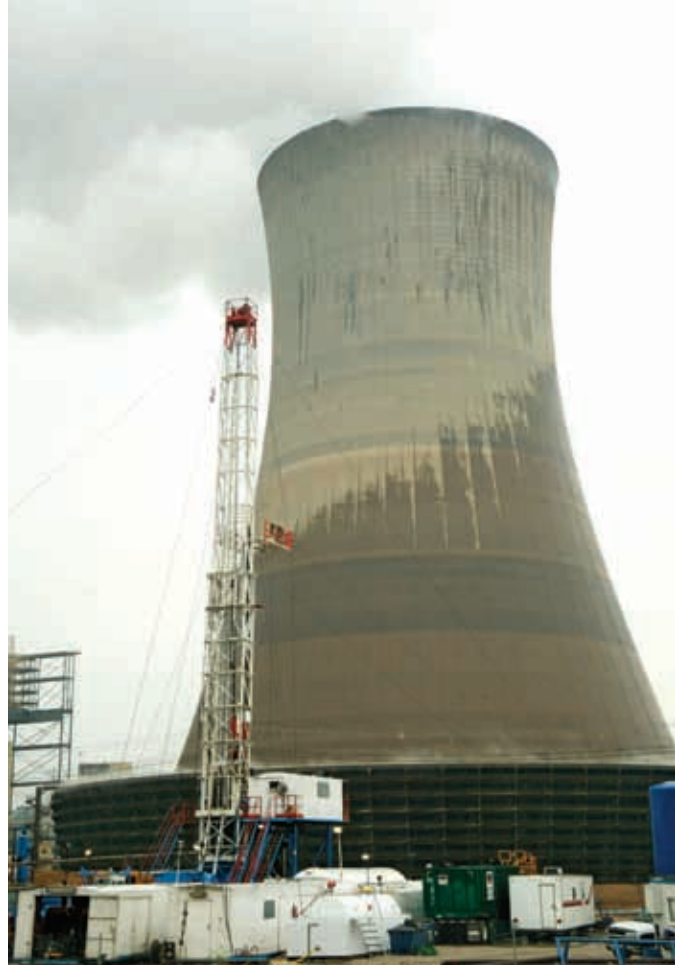
▲ Battelle researchers drill a 9,200-foot-deep sequestration test well at an American Electric Power generating plant in New Haven, W.Va.
