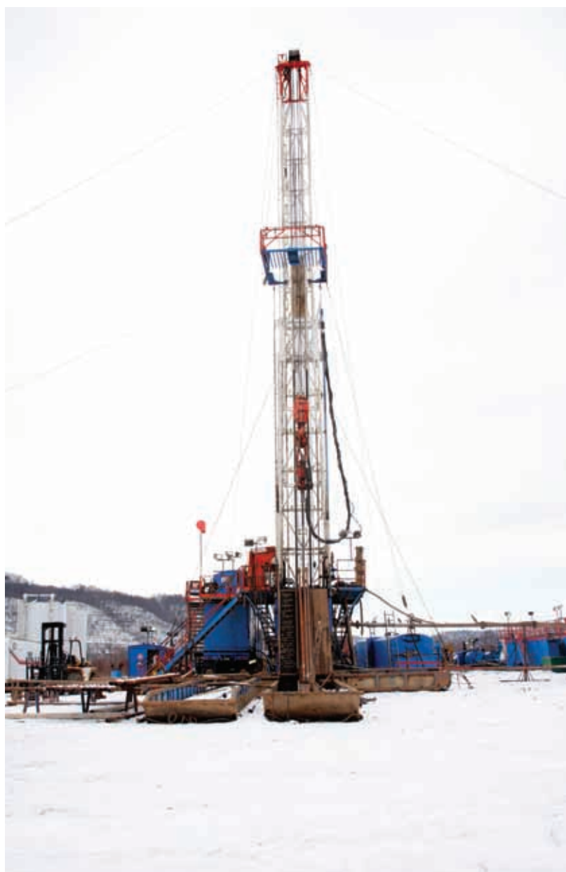
▲ Battelle researchers drill a 9,200-foot-deep sequestration test well at an American Electric Power generating plant in New Haven, W.Va.
