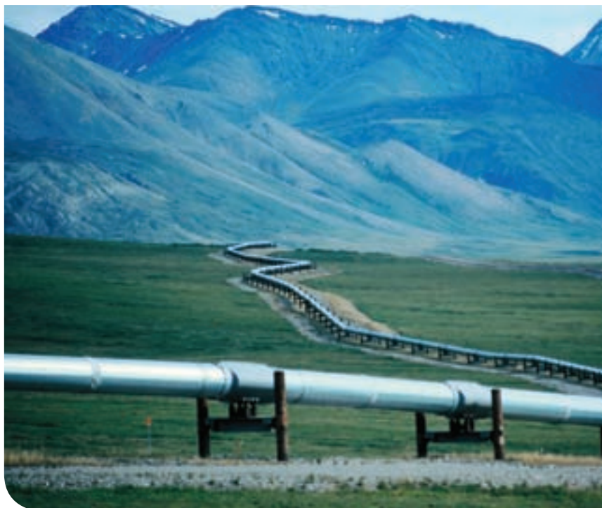
When the Clean Air Act of 1990 passed, natural gas was labeled the "fuel of choice."
