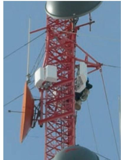
A radio node supports two-way wireless communications with substation equipment. PHOTO COURTESY OF ARCADIAN NETWORKS
