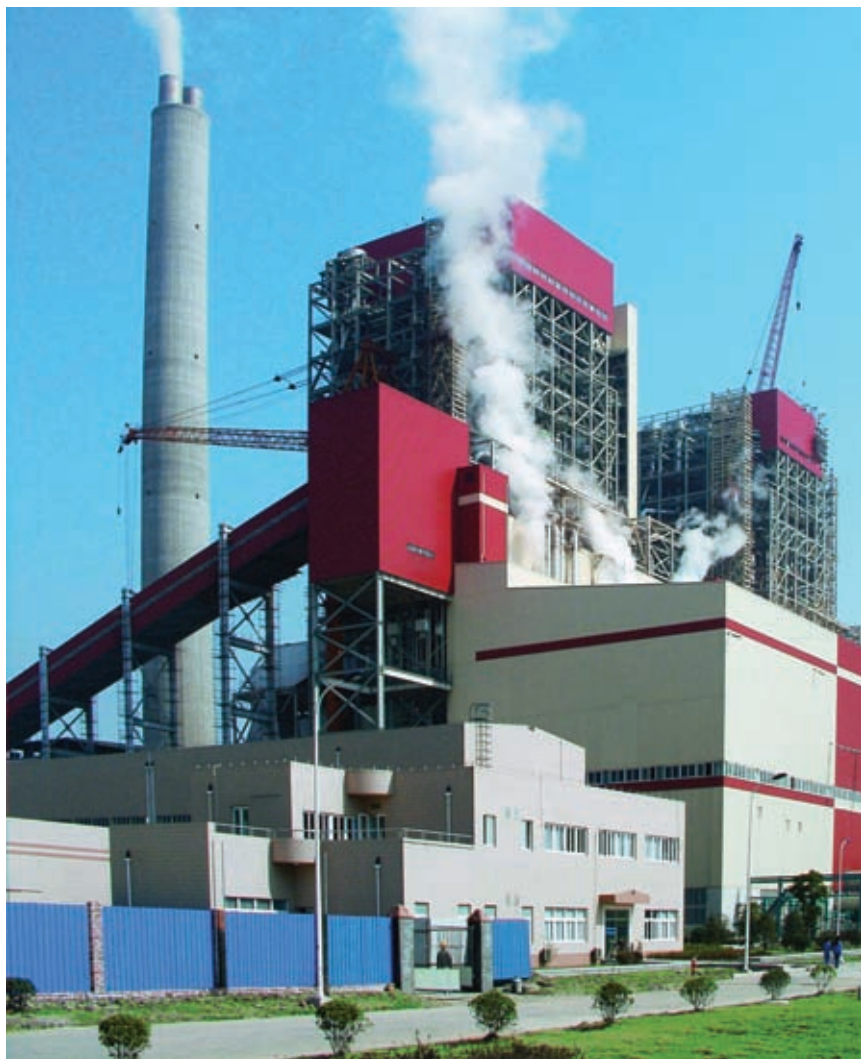
China is rapidly adding new coal-fired generation plants, including the Waigaoqiao plant located in Pudong, Shanghai, which provides 40 percent of Shanghai's power. The $1.9 billion plant opened in 2004.
