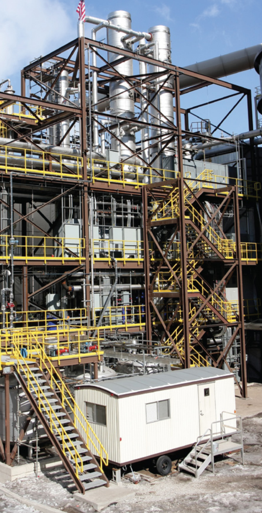
The 1.7-megawatt carbon-capture pilot project at We Energies' Pleasant Prairie, Wis., plant. PHOTO COURTESY OF WE ENERGIES
