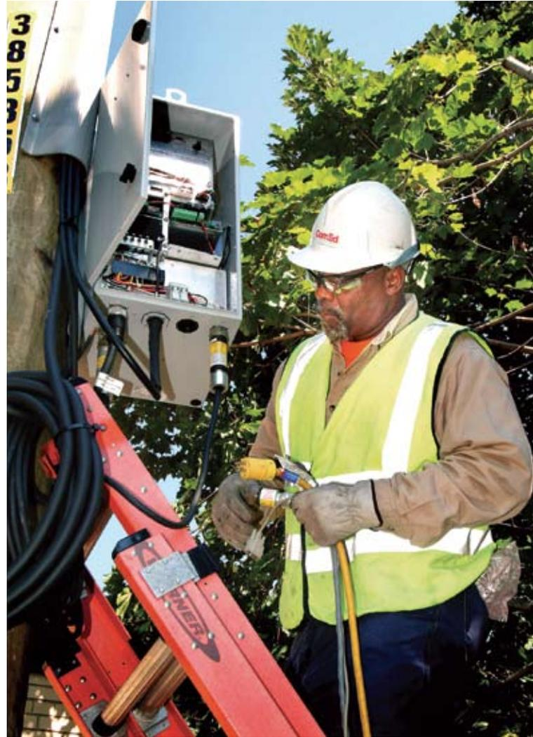
▲ Chuck Brown, a principal technician with ComEd distribution testing, tests the controller cabinet near a recently installed midcircuit reclosure on Chicago's North Side.
